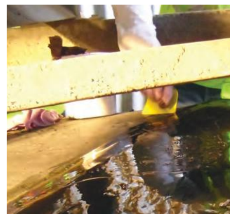
After Repair: Belt flap cut down, Devcon Surface Conditioner and R-Flex applied to belt.
